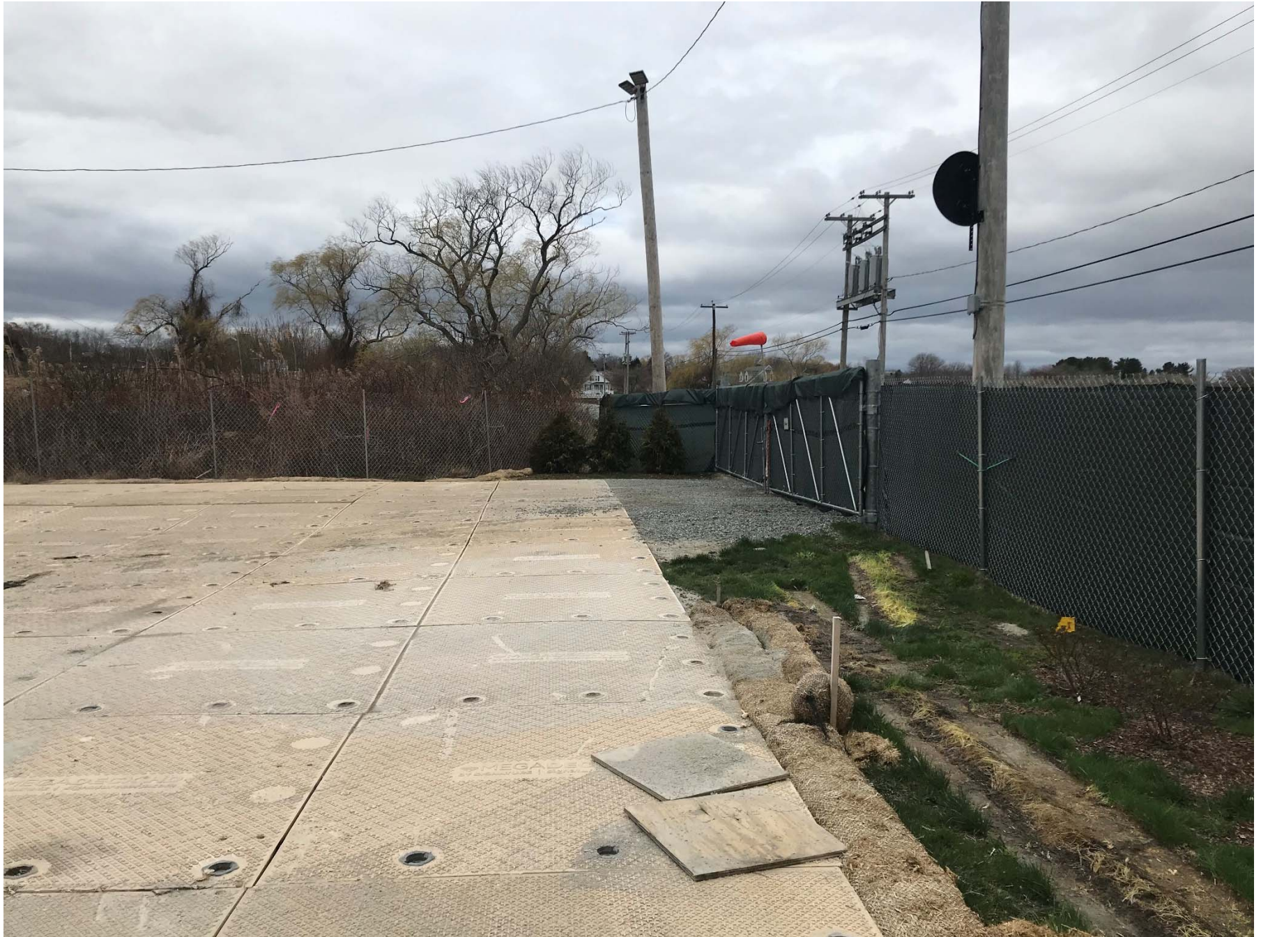
Photo of Fences and Temporary Mats
