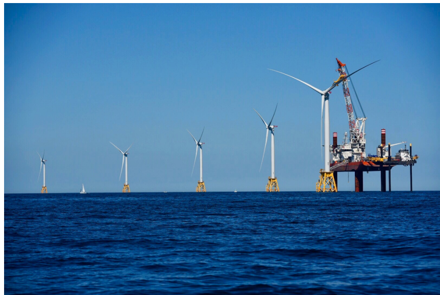
Figure 10-5: Installation of the Final Blade at BIWF
