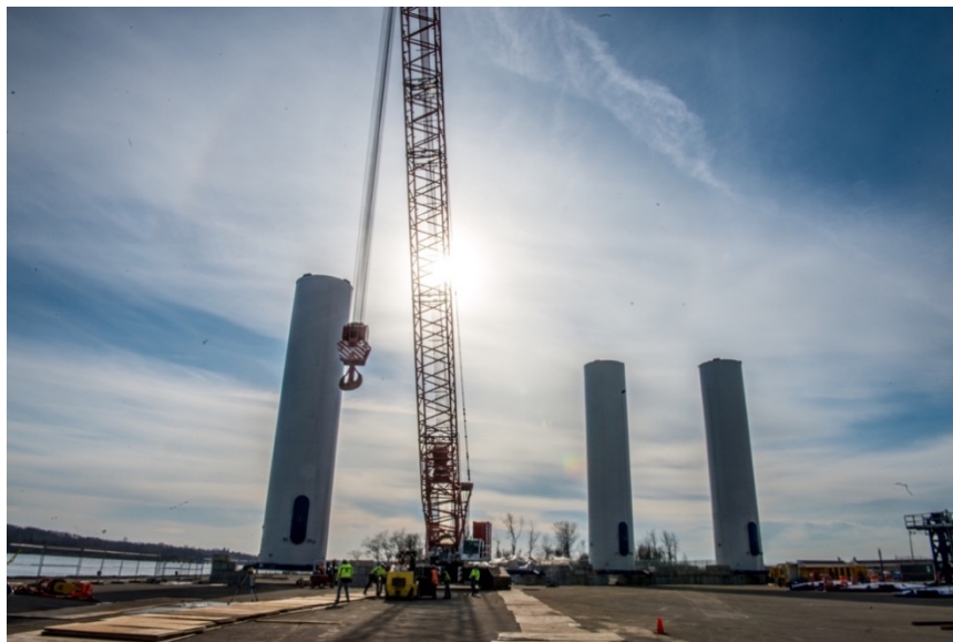
Figure 10-1: BIWF Turbine Assembly at the Port of Providence (RI)
