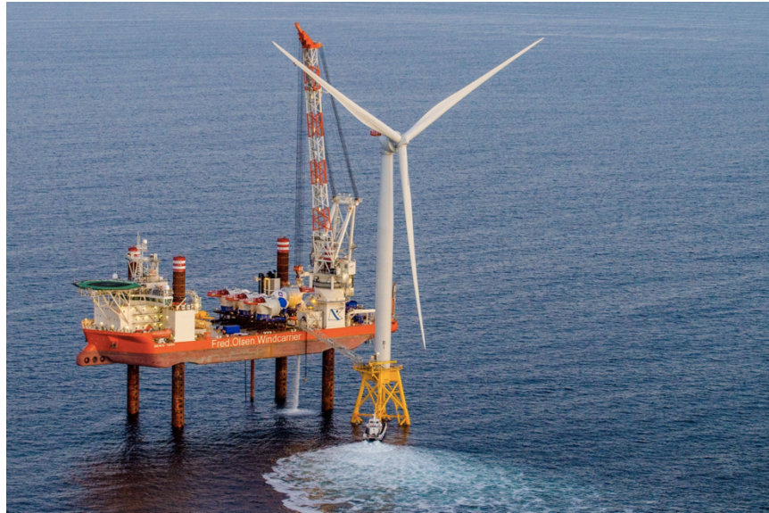
Figure 10-4: Installation of First BIWF WTG
