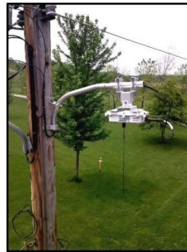
Figure 5.3: Pole-Mounted Network Equipment
