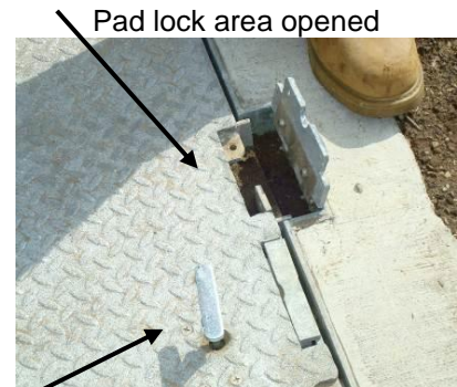
Recessed pad lock area Hatch opening lock Hatch bolts
