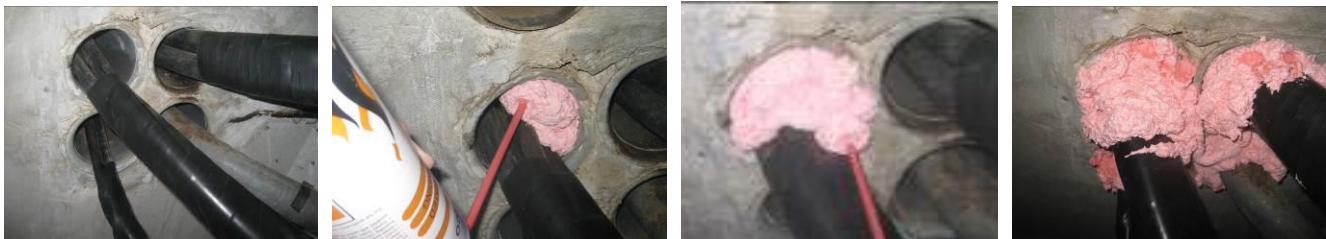
Fire-stop sealant installation
