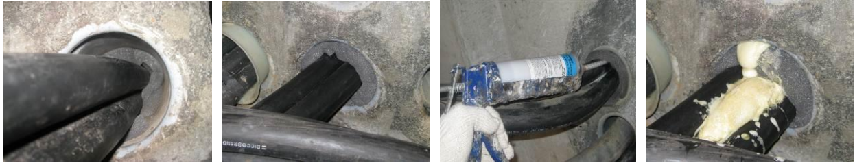
Water stop sealant installation
