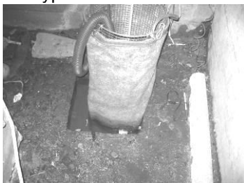
Filter set into sump hole
