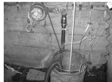
Sump discharge hose installed to drain and filter basket bonded.
