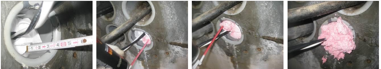
Fire-stop sealant installation
