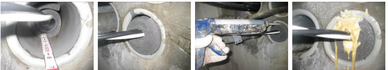
Water stop sealant installation
