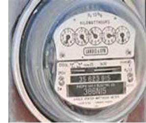
Electro-mechanical Meter
