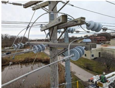
Figure 2 Pole 6 Beach Avenue Access Road
