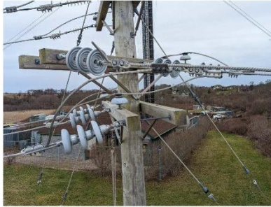
Figure 1 Pole 5 Beach Avenue Access Road
