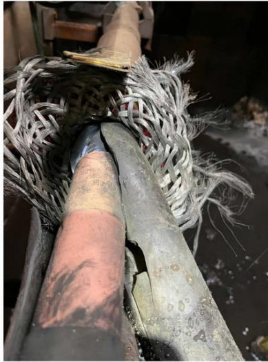
Figure 2 MH 9024 Point Judith Road
