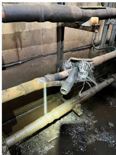
Figure 1 MH 9024 Point Judith Road
