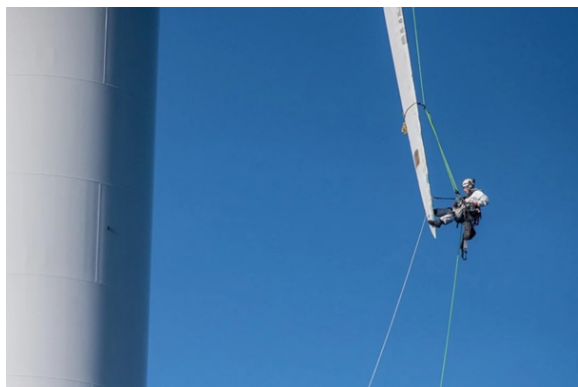
Fancher inspects the turbine blade’s tip receptor. Neil Ever Osborne
