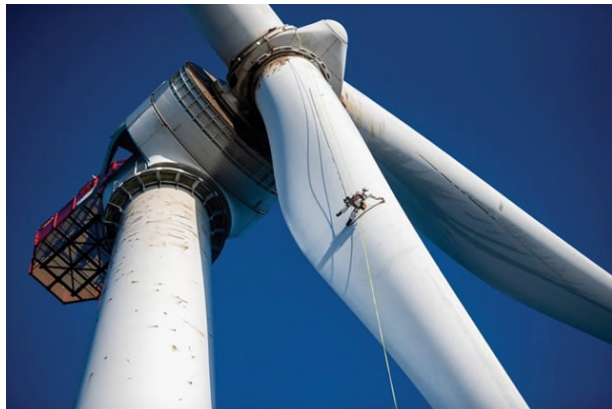
Hundreds of feet above the sea, Will Fancher, a rope access supervisor for the Block Island Wind Farm, performs maintenance that is far from routine. Neil Ever Osborn
