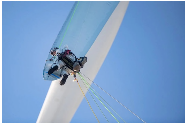
Fancher working on the turbine blade’s tip receptor. Neil Ever Osborne
