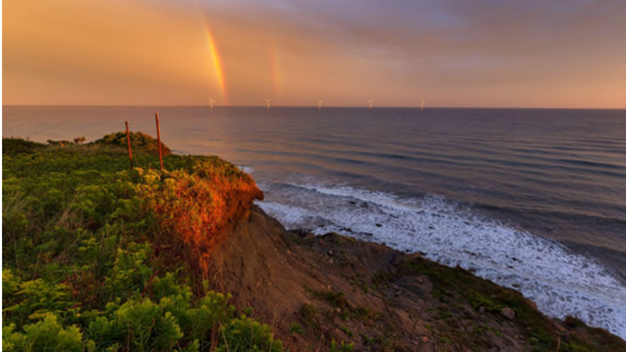
A rainbow illuminates the sky above Deepwater Wind's five turbines in the water off Block Island. (Aleksander via Chime In)
