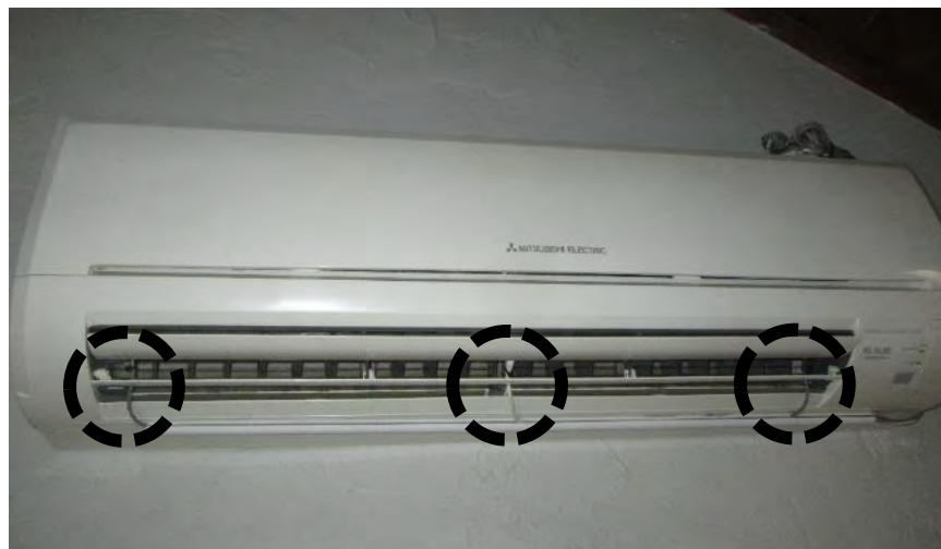
Figure 9. Leaving Air Sensors on a DMSHP Head
