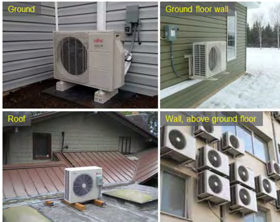
Figure 1. Outdoor Installation Types
