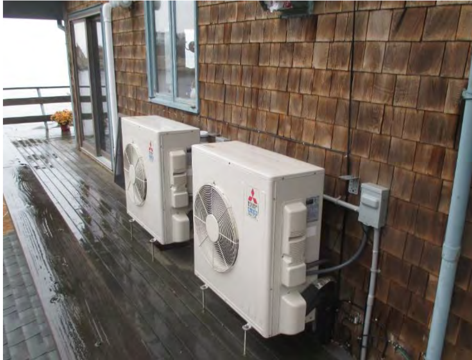
Figure 75. DMSHPs in Windy Environment
