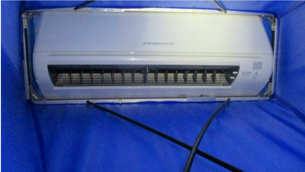
Figure 93. Non-Powered Flow Hood (Balometer) Setup
