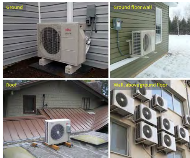
Figure 13. Outdoor installation types
