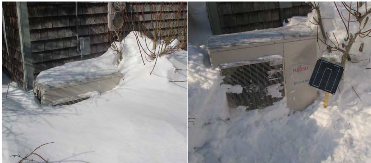
Figure 74. Maintaining Clearances in Wintertime
