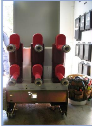
2011 Installation of Replacement
