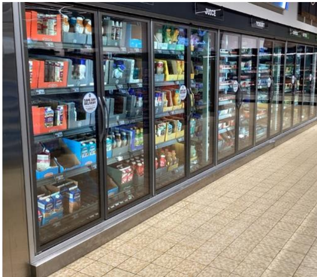
New lids on low temperature coffin cases and no heat doors for low and medium temp cases.
