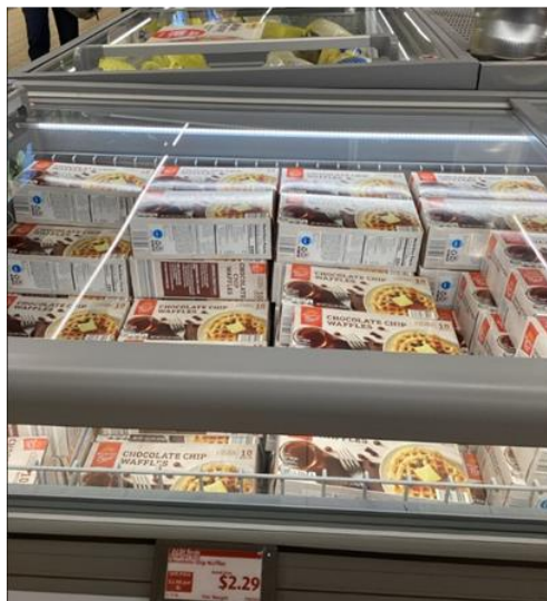
New lids on low temperature coffin cases and no heat doors for low and medium temp cases.
