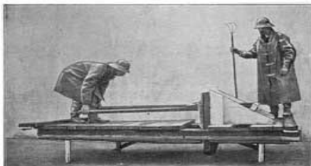
FIG. 7.—SCRAPER FOR LARGE SEWERS.
