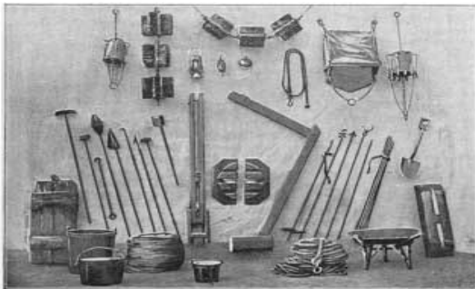
FIG. 3.—TOOLS FOR REMOVING OBSTRUCTIONS.
