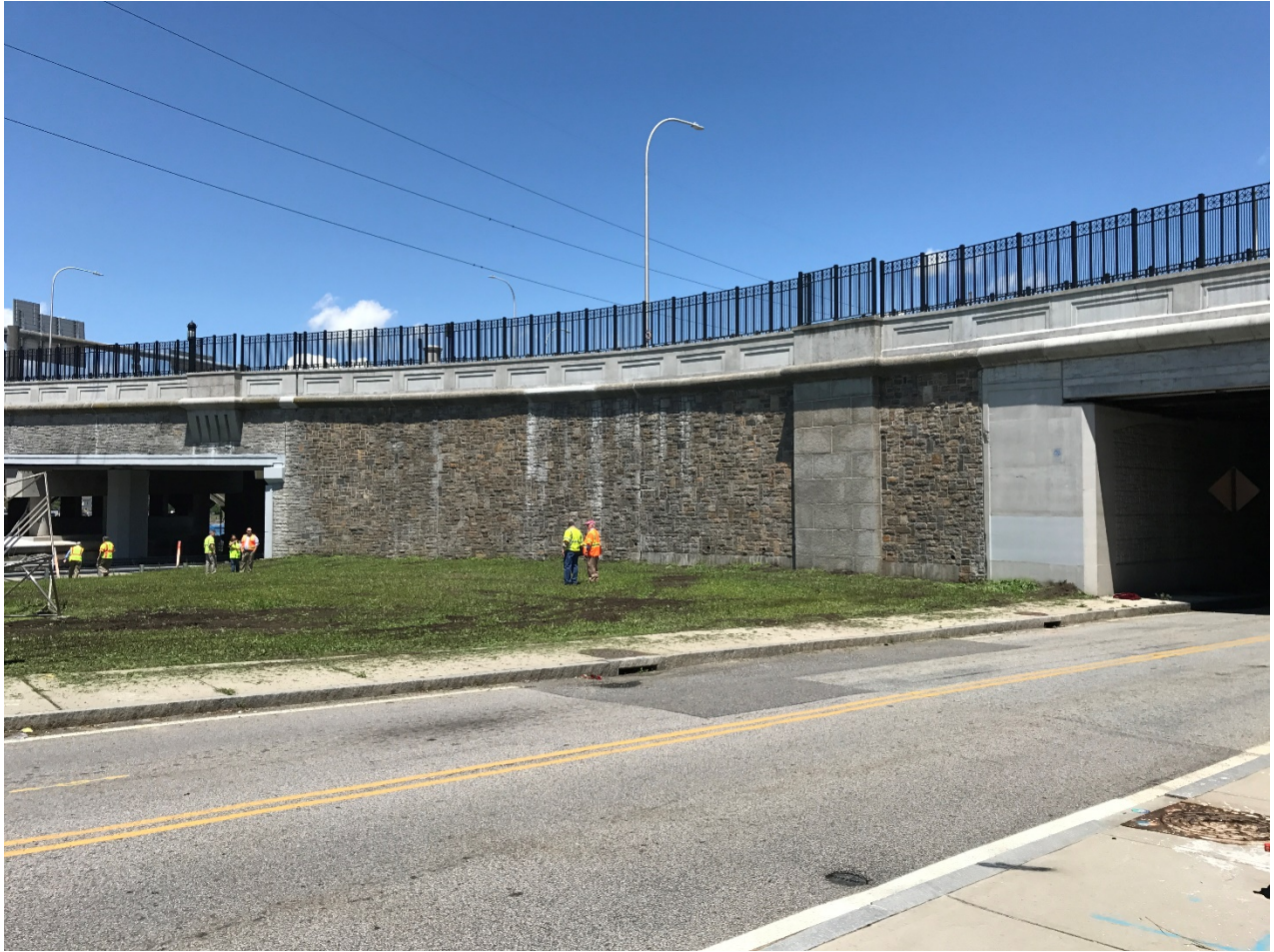
Figure 11 – Area between Bridges Requiring Open Cut Trenching
