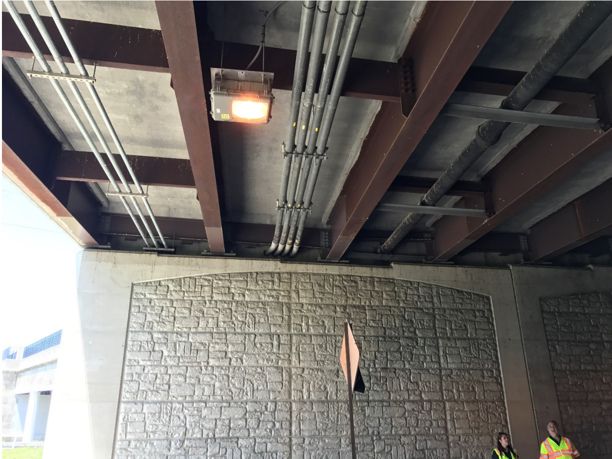
Figure 10 – Distribution or Street Lighting Circuits and Storm Water Drains Attached to the Water Street and Waterfront Drive Bridges
