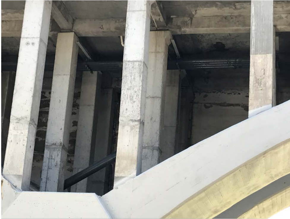
Figure 9 – Distribution or Street Lighting Circuits and Storm Water Drains Attached to Arch Portion of Bridge
