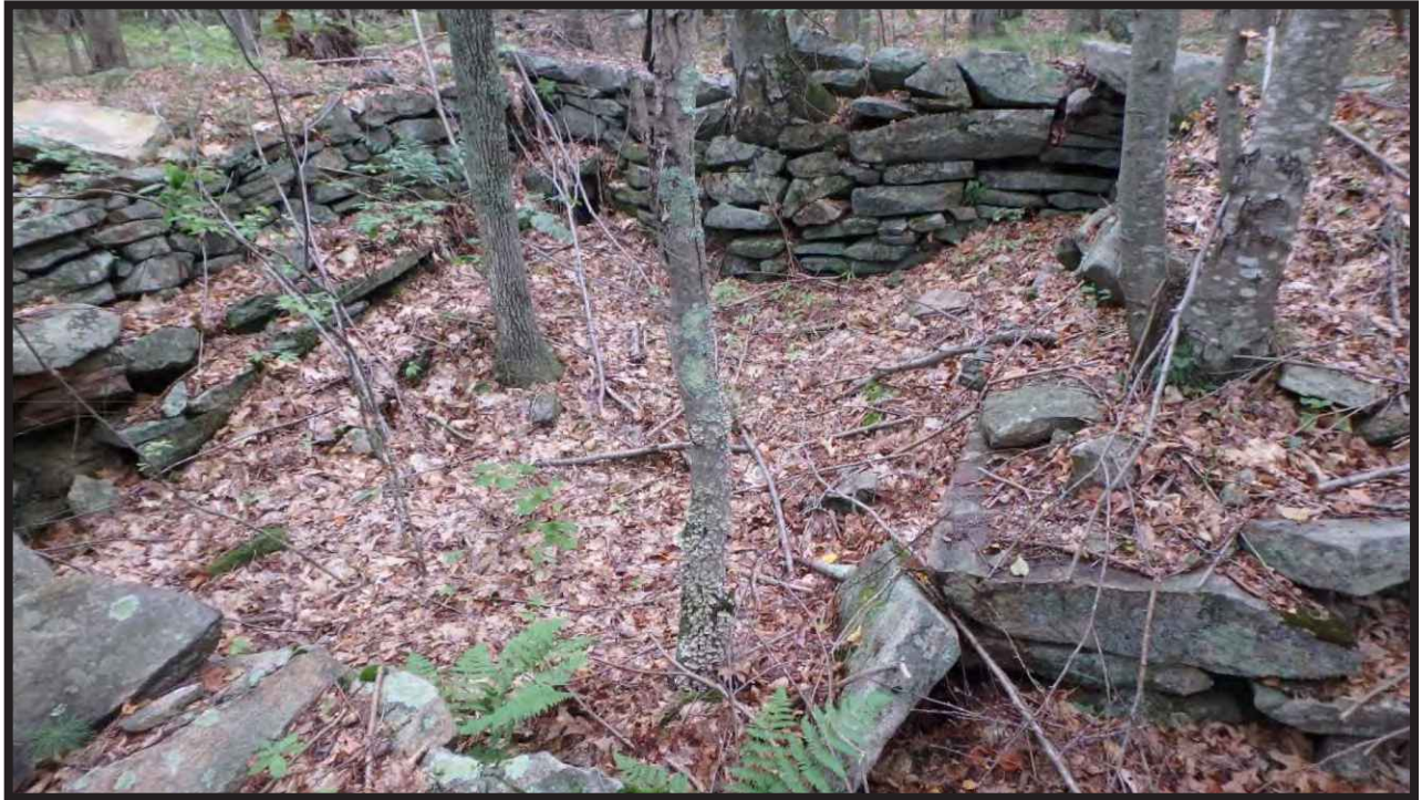
Plate 2. Dry-laid, stacked, stone foundation found along 345 kV line (2,500 feet).
