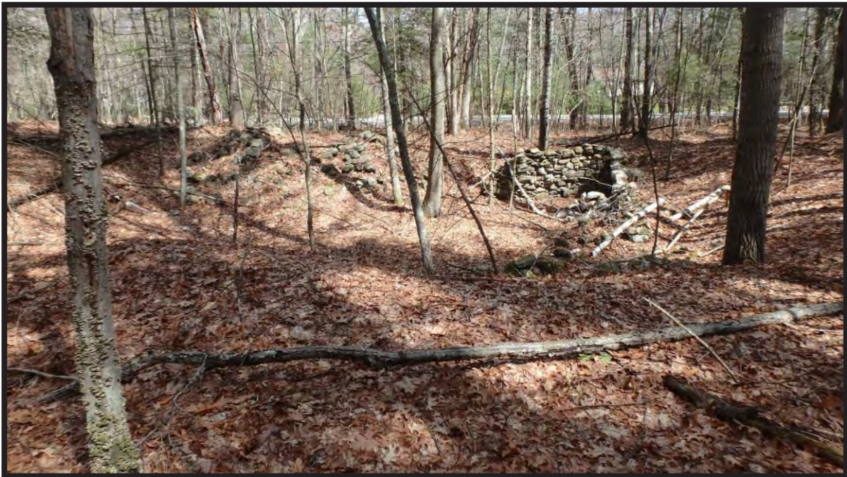
Plate 15. Dry-laid stone foundation identified in the northeastern portion of the Frontage Survey Area, view to the southeast.
