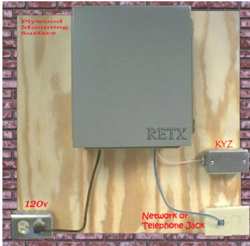
\* Maximum total run of 500 feet for KYZ pulses from meter to RETX box.
