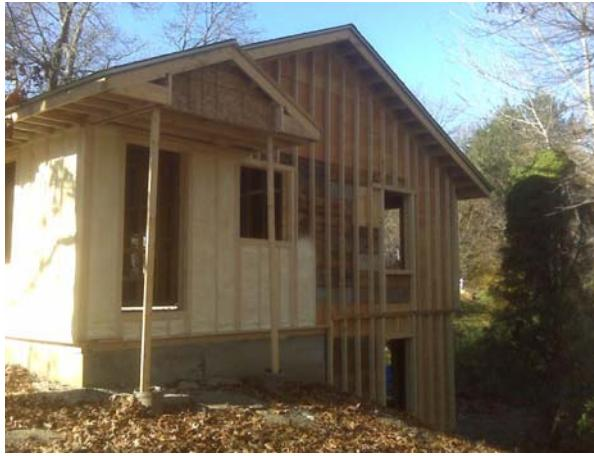
Exterior showing new exoskeleton with closed cell foam
