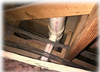
Plumbing/Wire Penetrations (before)
