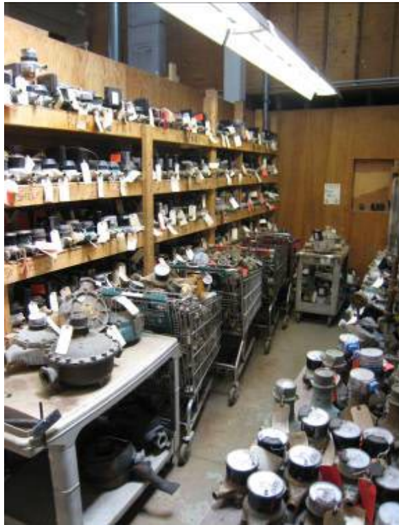
Providence Meter Room
