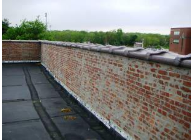
Providence Roof Wall
