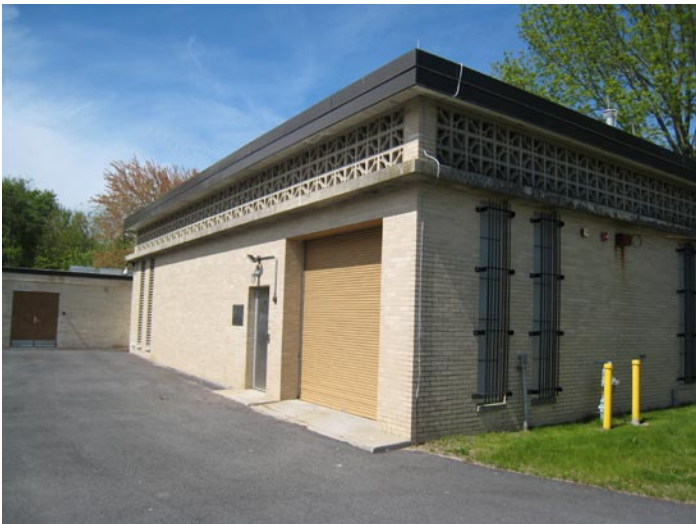
Cranston Pump Station/Records Storage
