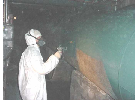
Recoating of 48" dia pipe in progress
