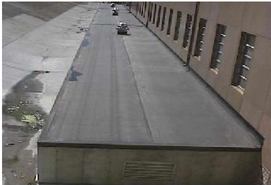
Completed clearwell protective structure
