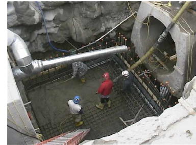
Pouring base slab of new valve enclosure
