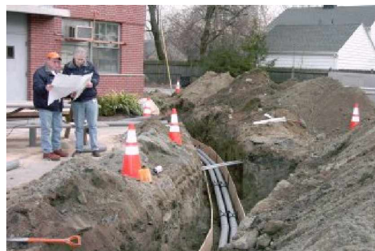
Excavation for Electrical Service to Academy Avenue
