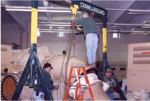
Installation of spool piece after valve installation
