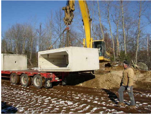
Unloading of culvert sections for residual management system
