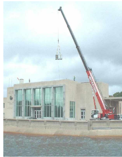
Placing A/C unit on top of the Auditorium
