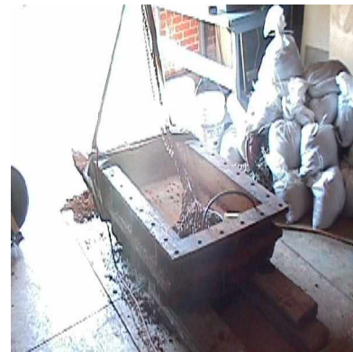
Old Longview Reservoir sluice gate being removed
