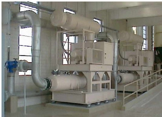
New air blower system at treatment plant for air scour backwashing of filters
