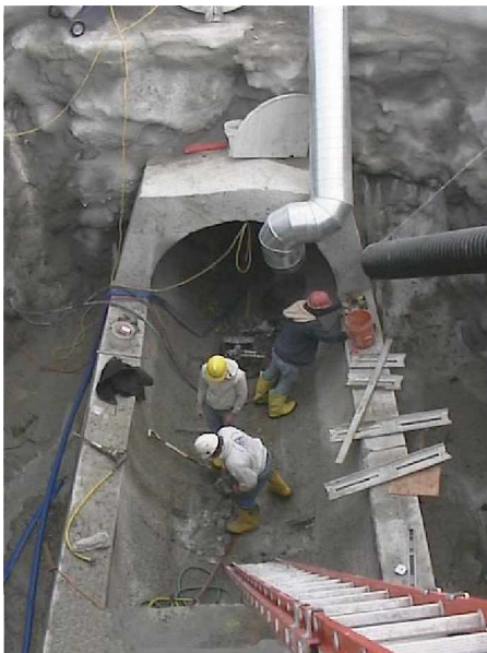
Access into 90" aqueduct at new valve location
