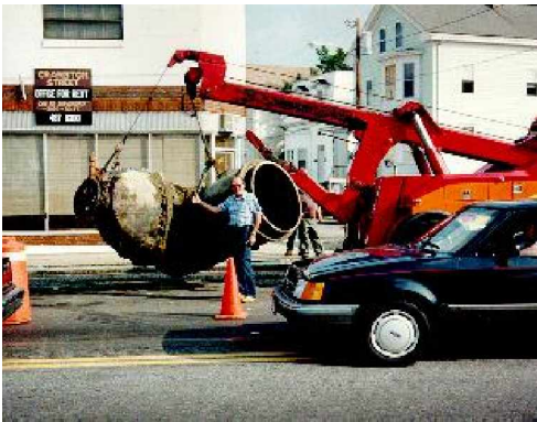
Removal of old 42 inch transmission gate valve
