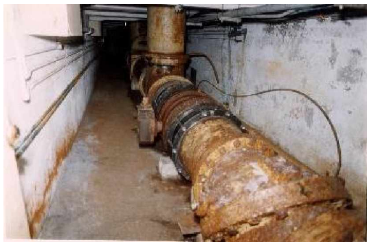
Neutaconkanut Pump Station piping before rehabilitation
