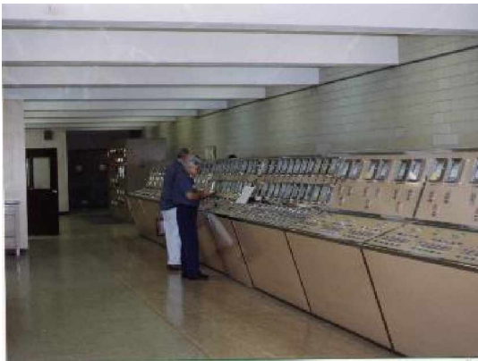
Old analog Central Control Board at treatment plant
