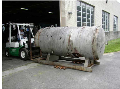
Removal of Original Forestry Boiler
