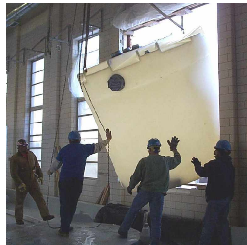
Bringing new Fluoride Storage Tank into the Treatment Plant
