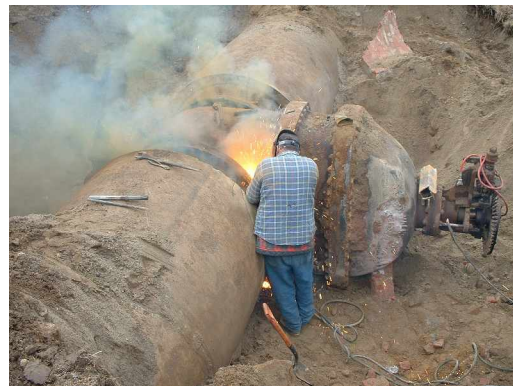
Removal of old 48 inch transmission gate valve
