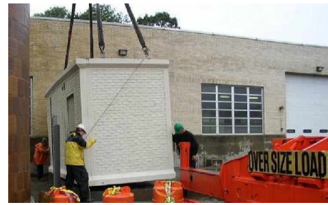
Lowering section of new blower building into place
