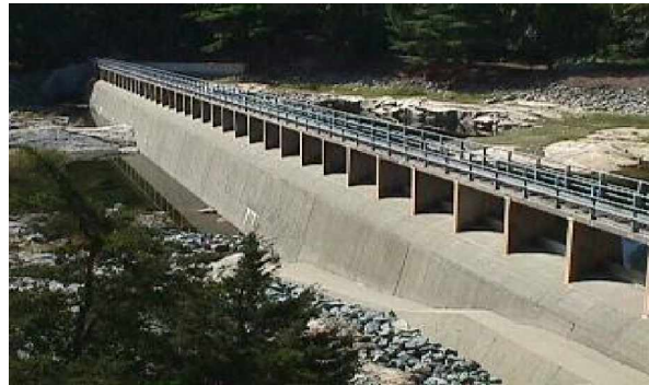
400 foot Gainer Dam spillway showing new concrete facing
