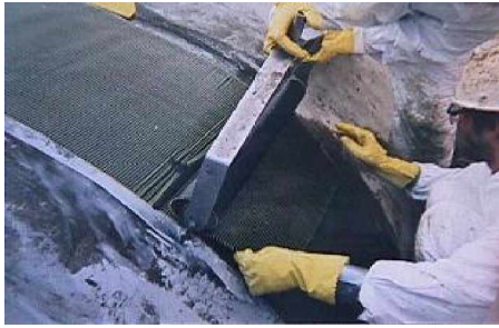
Application of carbon fiber to exterior of deteriorated section of 102" Aqueduct
