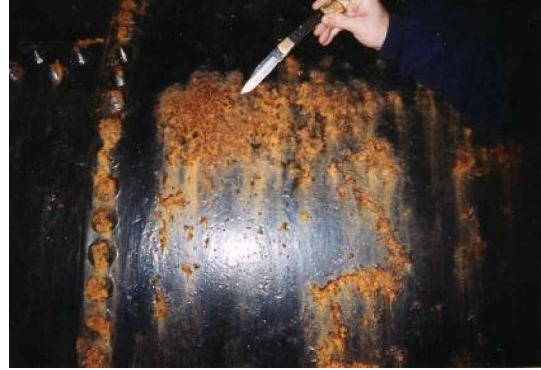
Corrosion on 60 inch main prior to rehabilitation
