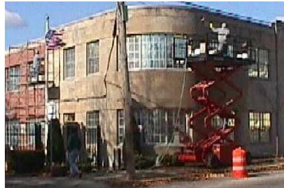
Restoration of the masonry and brickwork at Academy Avenue in progress
