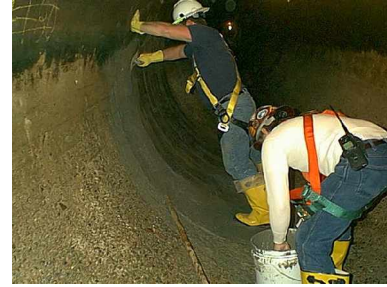
Concrete repairs to the interior of the 90" pipeline
