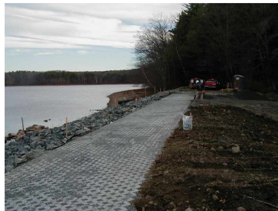
Regrading the access road on the crest of the dam
