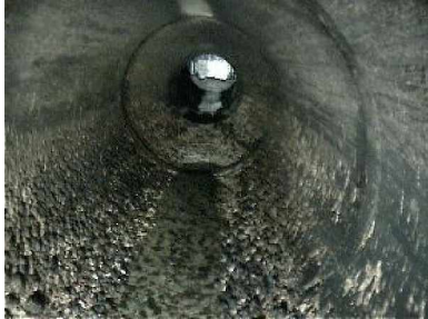
Concrete corrosion damage to the lower half of the effluent conduit
