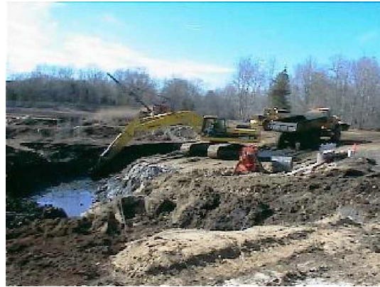
Sludge lagoon dredging operations in progress
