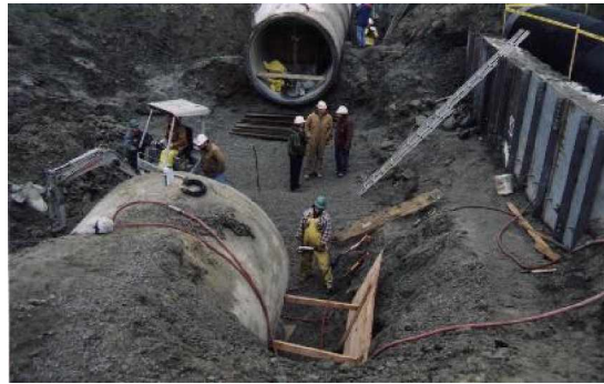
102" Aqueduct prepared for replacement sections
