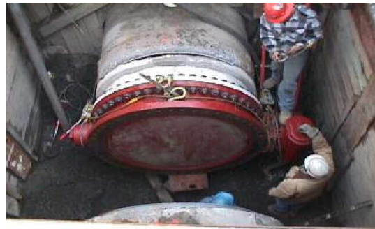
Installation of a new 60" butterfly valve to replace a defective valve at Budlong Road
