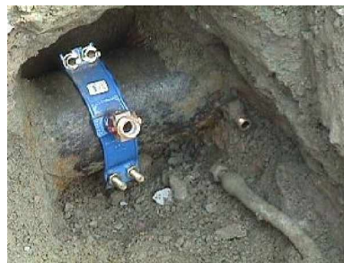
Typical lead service being replaced with a new copper service
