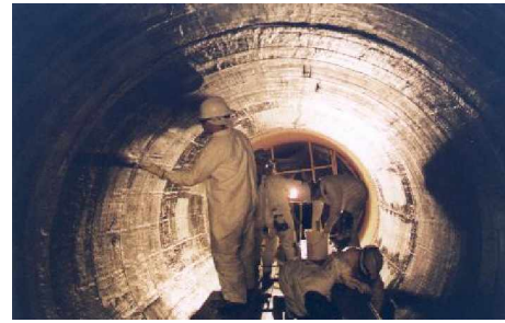
Crew applying carbon fiber lining to interior of deteriorated section of 102" Aqueduct
