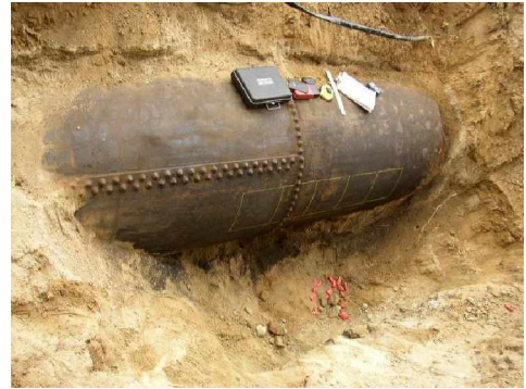
External section of 48" Washwater pipe
