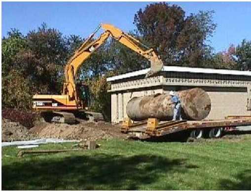
Removal of old underground fuel storage tank at the Aqueduct Pumping Station
