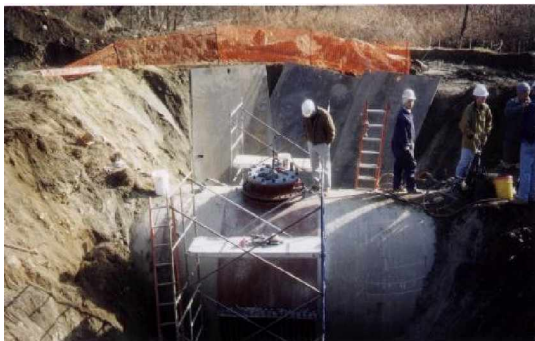
Installation of new access manhole into 102" Aqueduct
