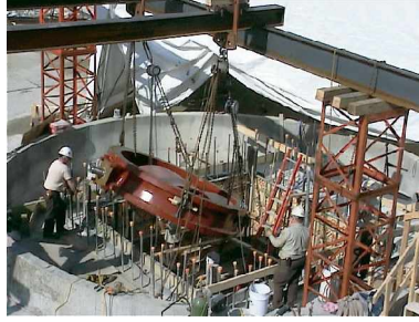
Lowering the 90” valve into place
