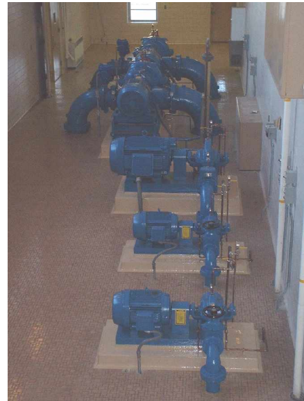
New Pumps following replacement
