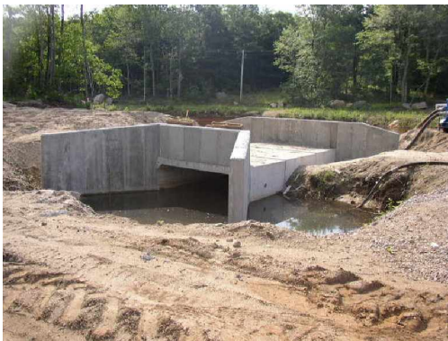
Culvert sections prior to backfill
