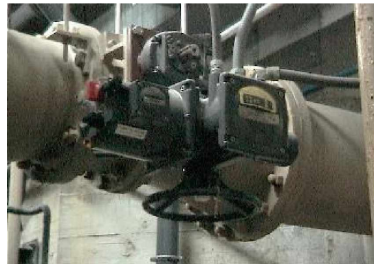
Typical new effluent valve actuator at treatment plant providing precise plant effluent control
