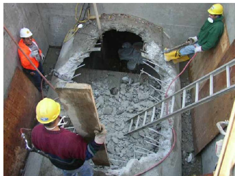
Opening into Aqueduct at New Access Structure
