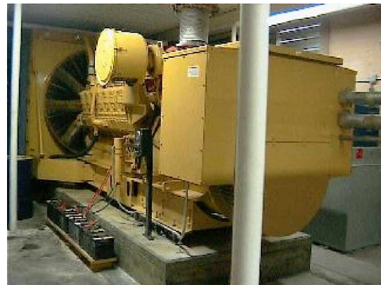
New Raw Water Booster Pump Station generator for backup power to treatment plant
