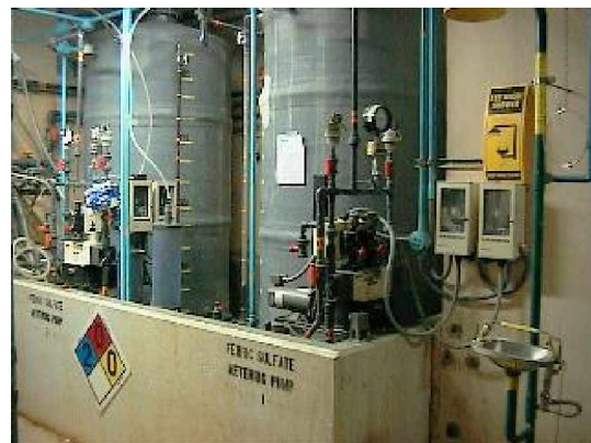
New sulfate feeder equipment and day tanks for liquid ferric sulfate coagulant injection
