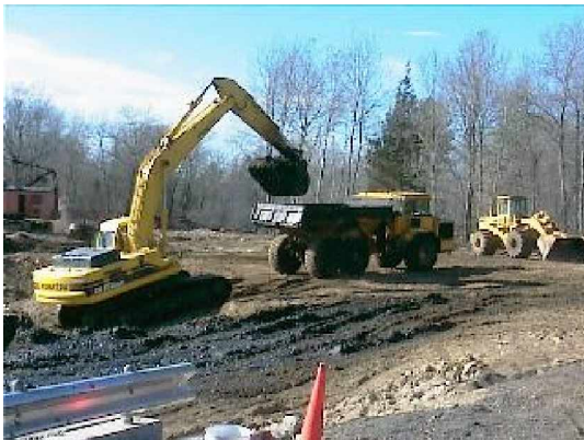
Sludge lagoon dredging operations in progress
