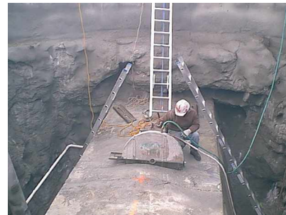
Sawcutting top of 90" pipeline to gain access for repairs and valve installation
