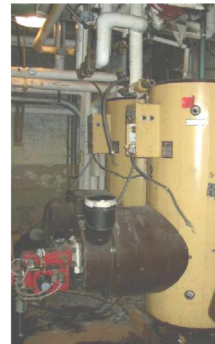
Old Process Water Heaters
