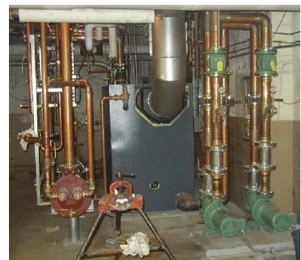
New Process Water Boiler
