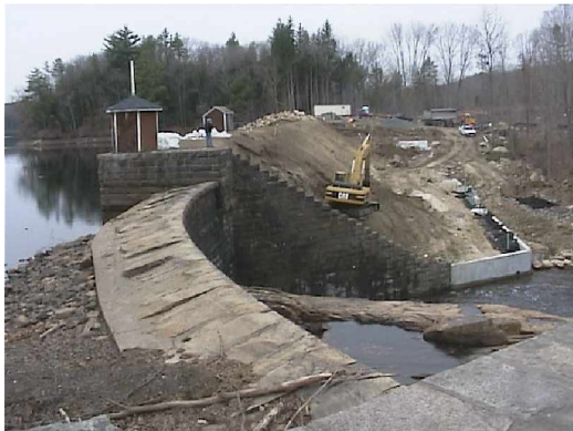
Repairs to the downstream slope of the dam
