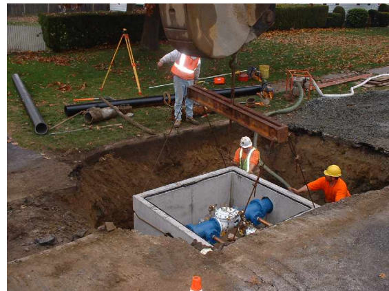
Installation of Pressure Reducing Valve Station
