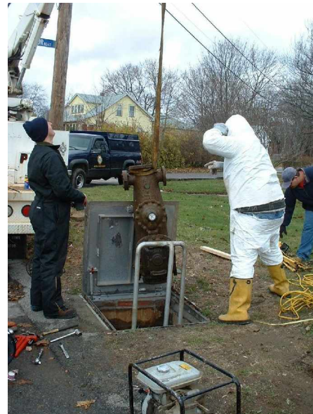
Removal of old meter from meter pit
