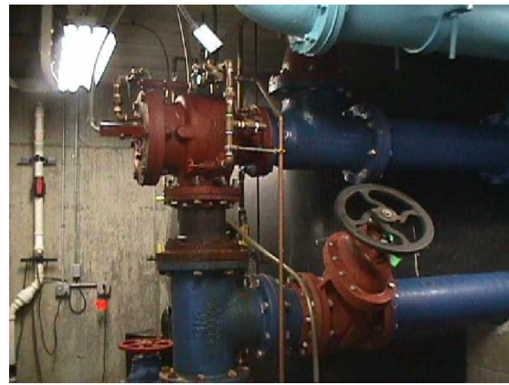
New surge control valve at Greenville Avenue Pump Station
