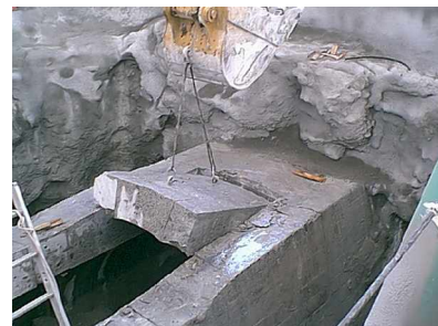
Removal of top of 90" pipeline
