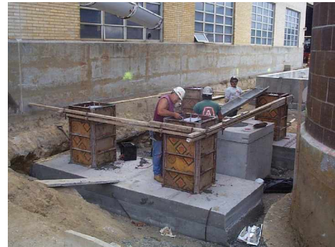
Footings for new access stairs to silos
