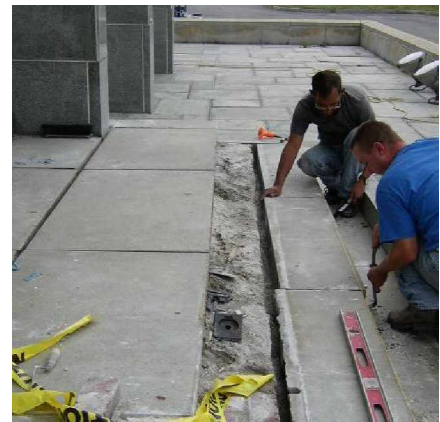
Resetting sections of stone on the stairs
