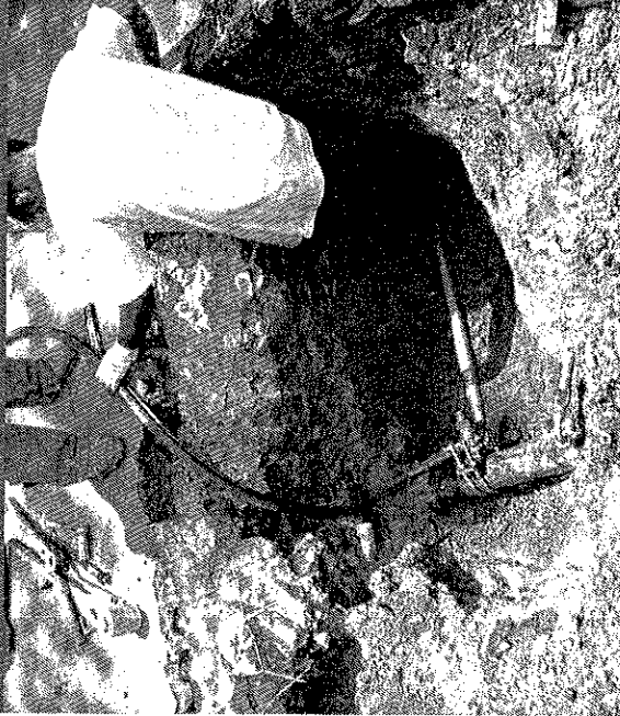
Contractor using trenchless technology (mole) for installing service line
