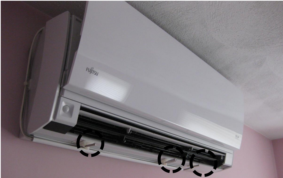
Figure 5. Leaving Air Sensors on a DMSHP Head
