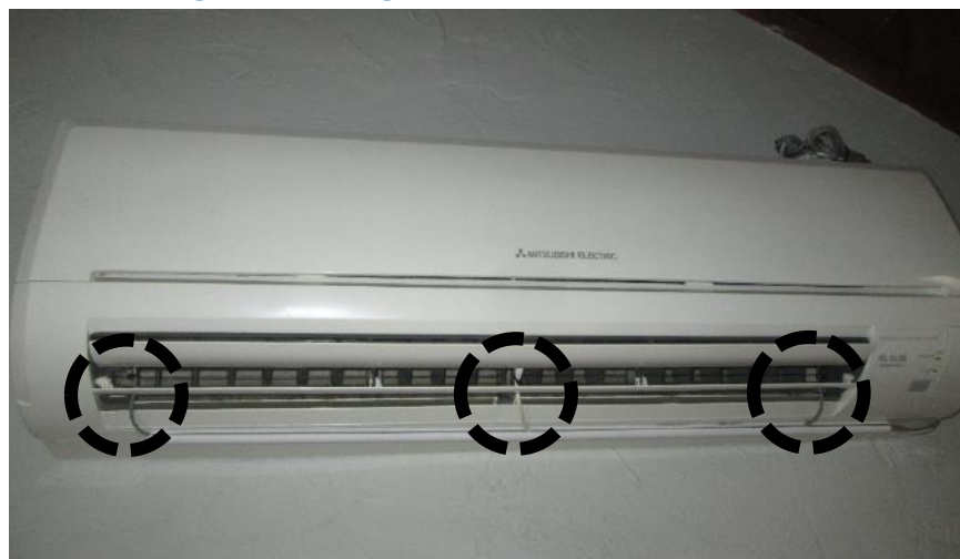
Figure 9. Leaving Air Sensors on a DMSHP Head
