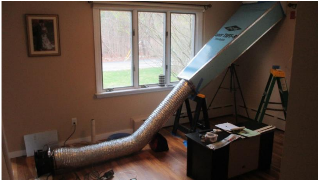
Figure 88. Powered Flow Hood Testing Setup
