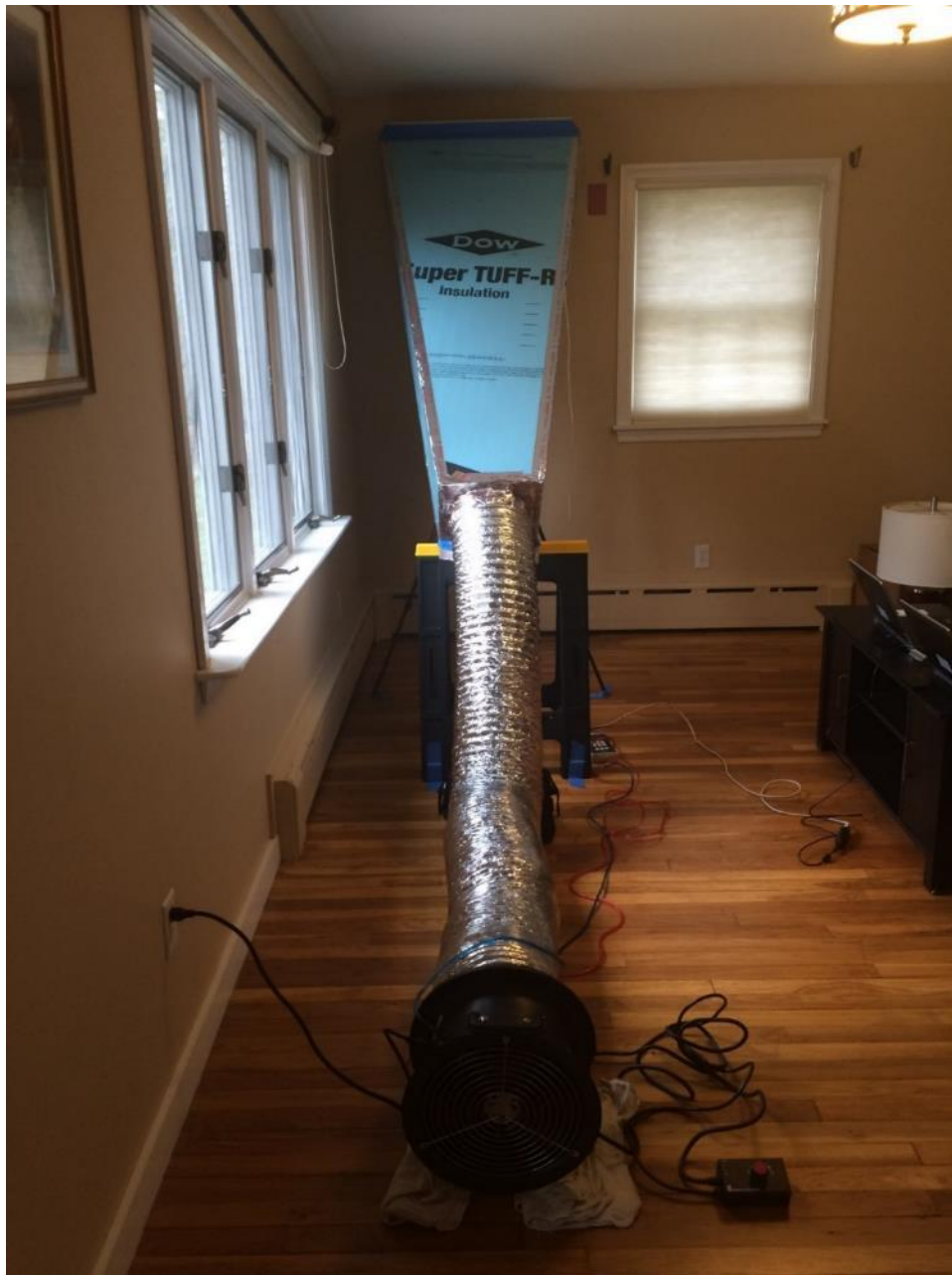
Figure 89. Powered Flow Hood Testing Setup
