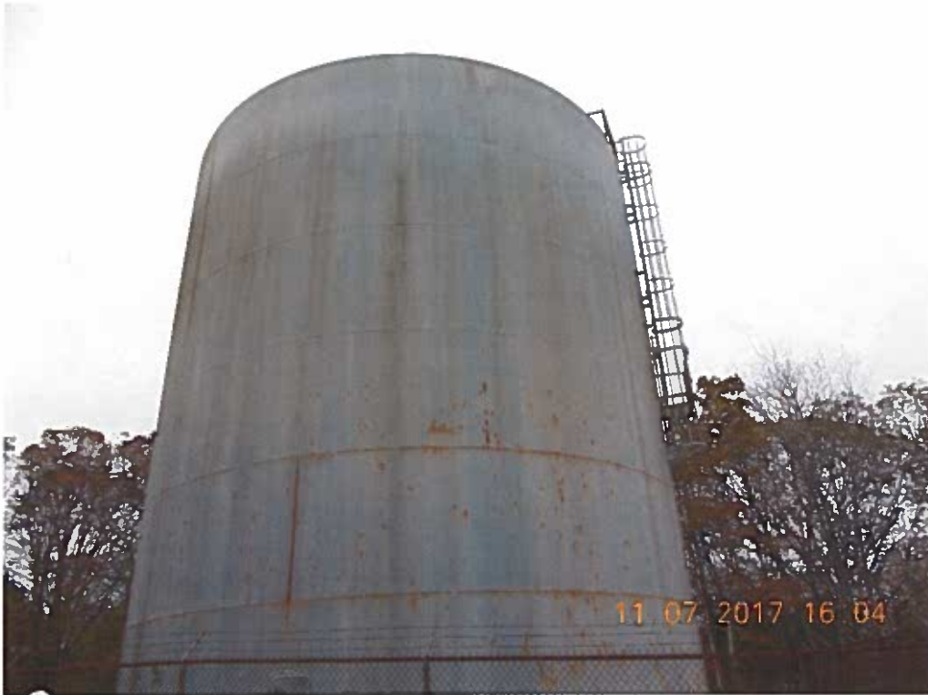
Account 330, Distribution Reservoirs and Standpipes Tank – Old – Standpipe
