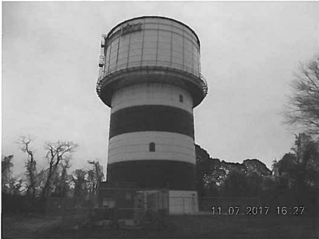
Account 330, Distribution Reservoirs and Standpipes Elevated Tank
