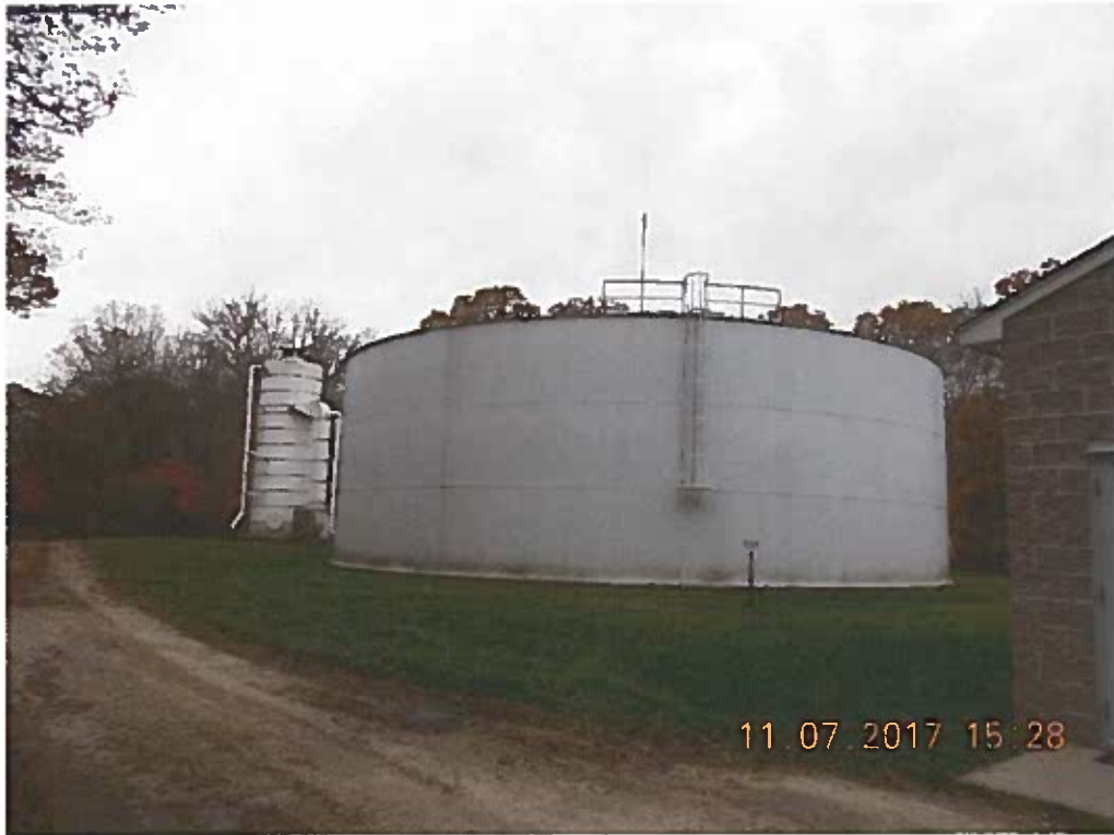
Account 330, Distribution Reservoirs and Standpipes Standpipe and Air Stripper
