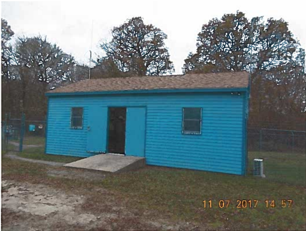
Account 304.1, Structures and Improvements - Source of Supply Pump Building
