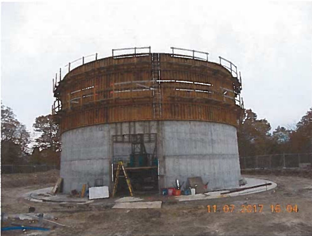
Account 330, Distribution Reservoirs and Standpipes Tank – New – Under Construction
