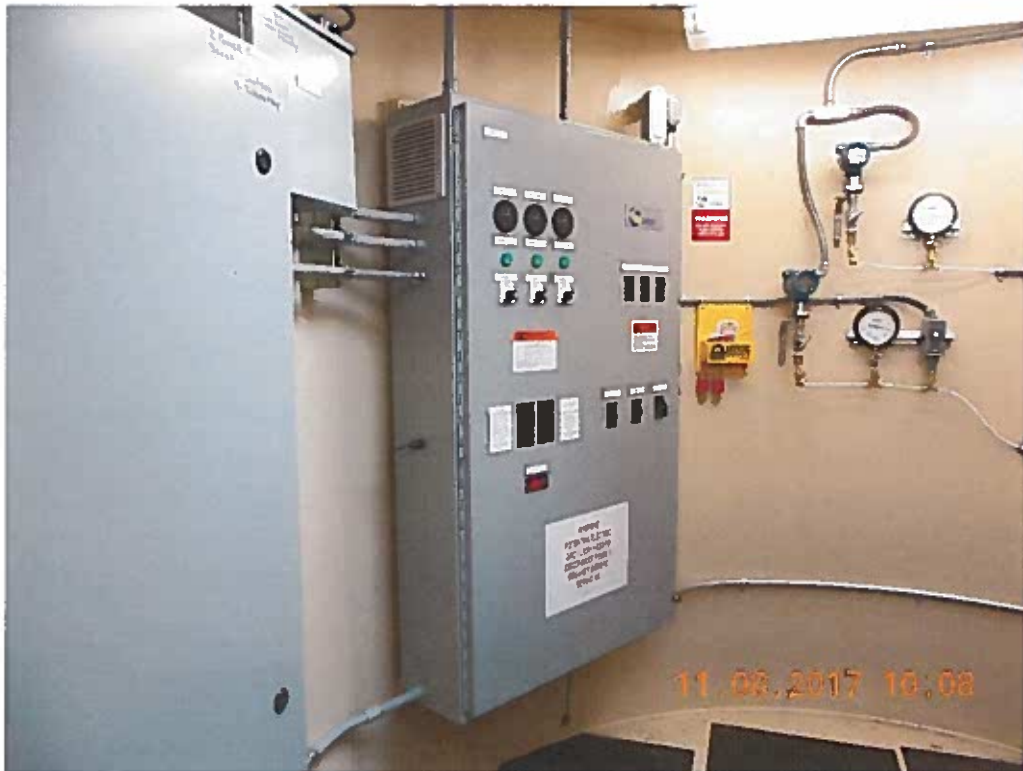
Account 304.1, Structures and Improvements - Source of Supply Controls
