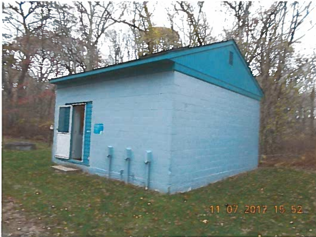
Account 304.1, Structures and Improvements - Source of Supply Well House
