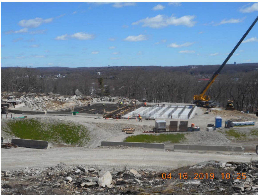
Chlorine Contact Tank - North Slab Reinforcement and Completed South Slab Concrete
