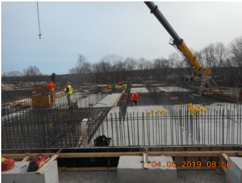
Chlorine Contact Tank - South Slab Reinforcement and Placement of Slab Sections
