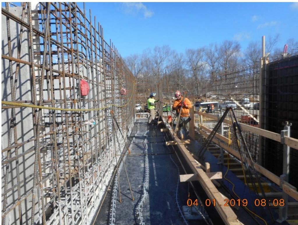
Process Building- Trough Slab Reinforcement
