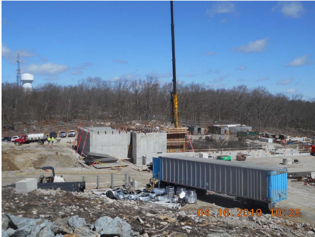
Process Building- DAF Walls Formwork and Reinforcement
