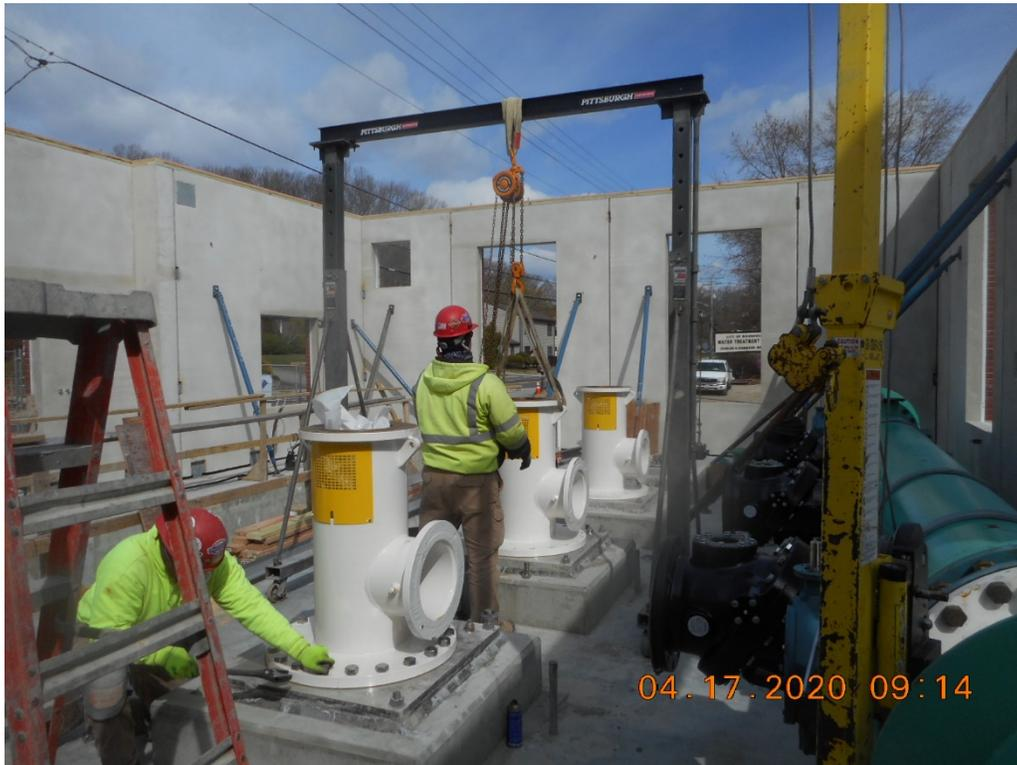
**Installation in Progress for RWPS Vertical Turbine Pumps**
