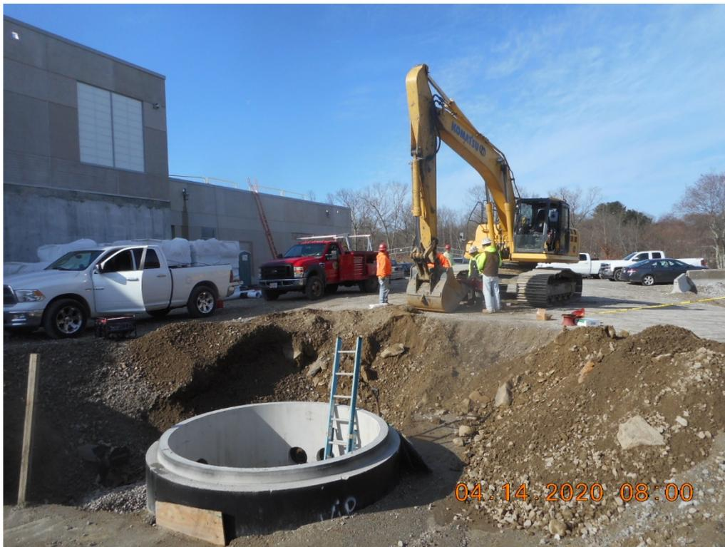
**Installation of Sanitary Wetwell at WTP**
