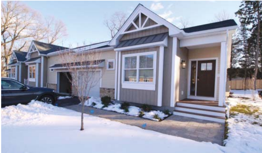
Pictured: First of the nine Wynfield Place homes. Grand Opening was December 2019.
