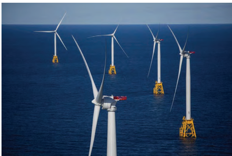
Figure 11-1: GE Wind Turbines Operating at Block Island
