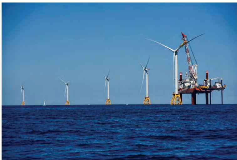
Figure 10-5: Installation of the Final Blade at BIWF
