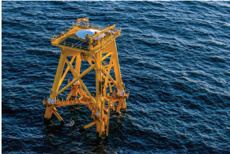
Figure 10-2: First BIWF Foundation
