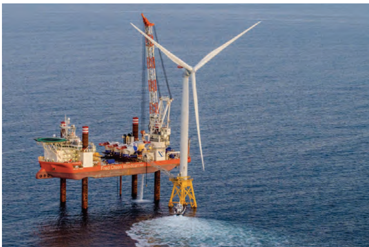
Figure 10-4: Installation of First BIWF WTG
