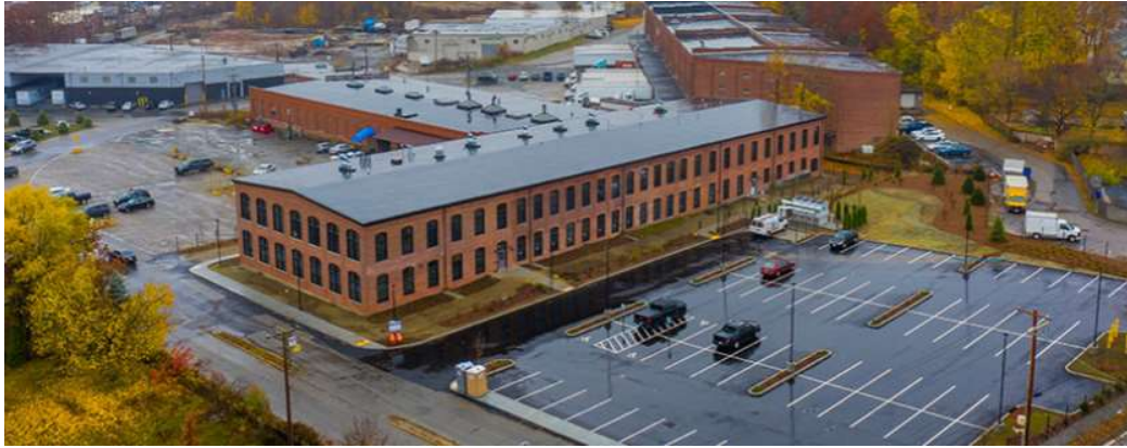
Pictured above: Lincoln Lofts, before and after renovation
