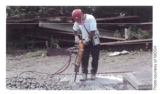
A worker chips concrete with a jackhammer using a water-spray attachment to control dust.
