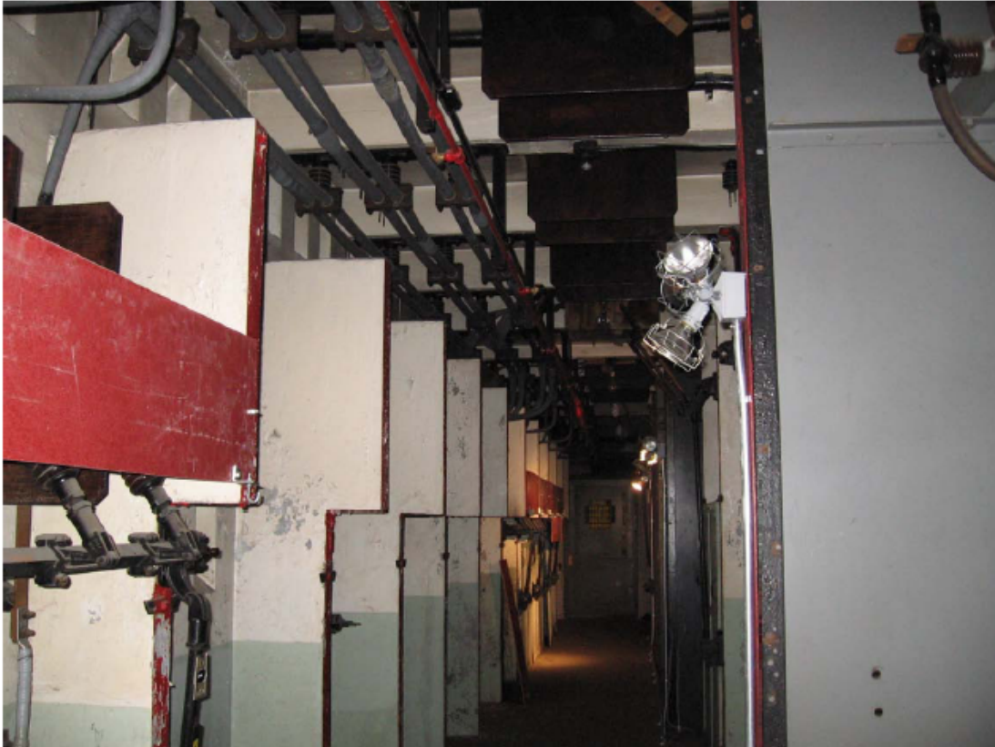
Room with 4.16kV -4 switches (left), -3 disconnects (ceiling)
