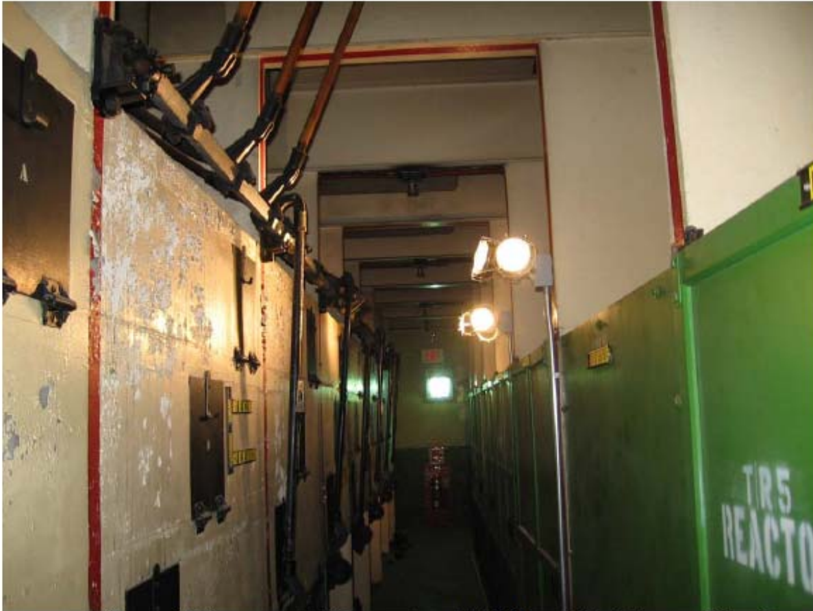
Room with Gang operated disconnects and 4.16kV bus – Black doors on left wall provide access to each phase energized bus. 1 of 2 such rooms
