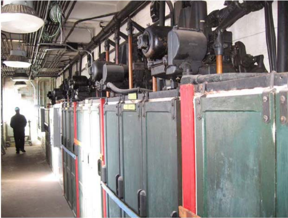
One of 7 Breaker Rooms with H-Type Breakers
