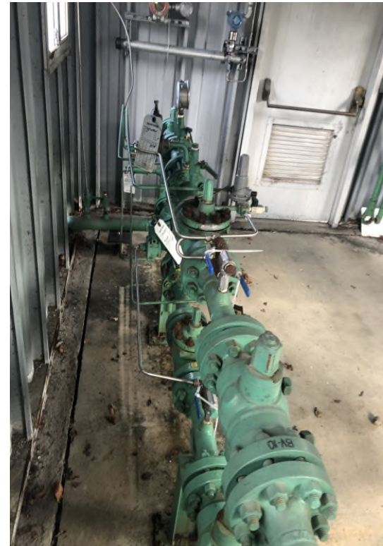
Two layer station with Fisher 399 and Grove 83 regulators pictured above which are both obsolete.
