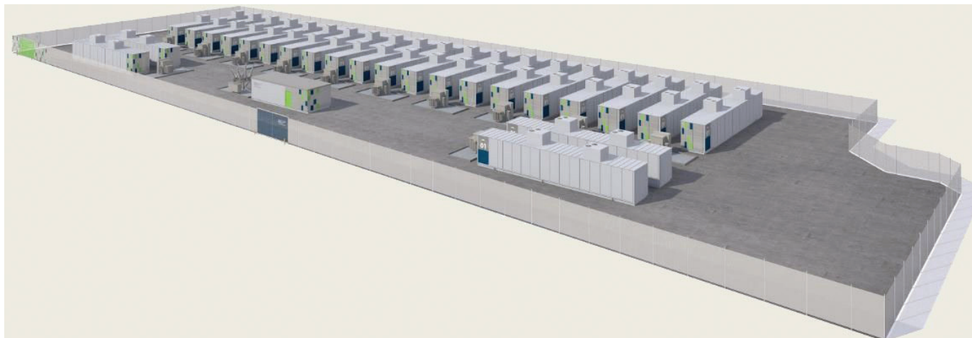
Figure 5: Typical 30 MW, 120 MWh Lithium-Ion Energy Storage Site 13
